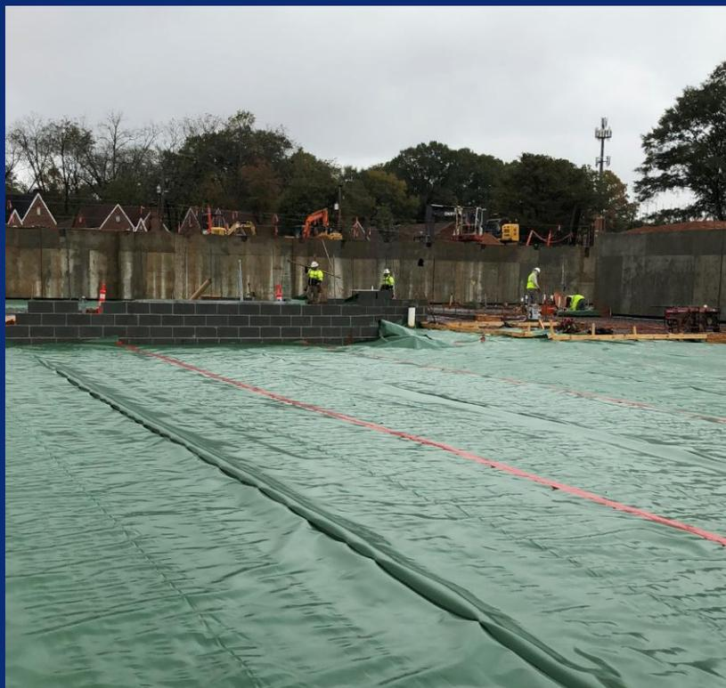
Lower level vapor being barrier installed for SOG pour
